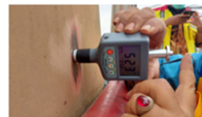
Fig 2b. Testing Girder
