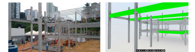
Fig. 10. Digital twin corresponding to the assembly process at the construction site.
